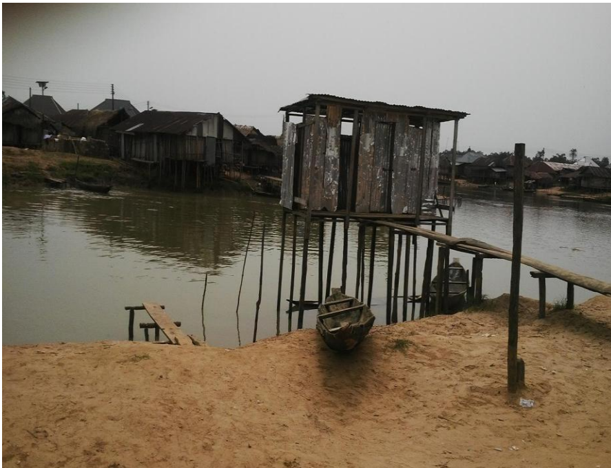
Plate 3: Showing a Toilet Building © O.K.Oyeoku & A.O.Angba
