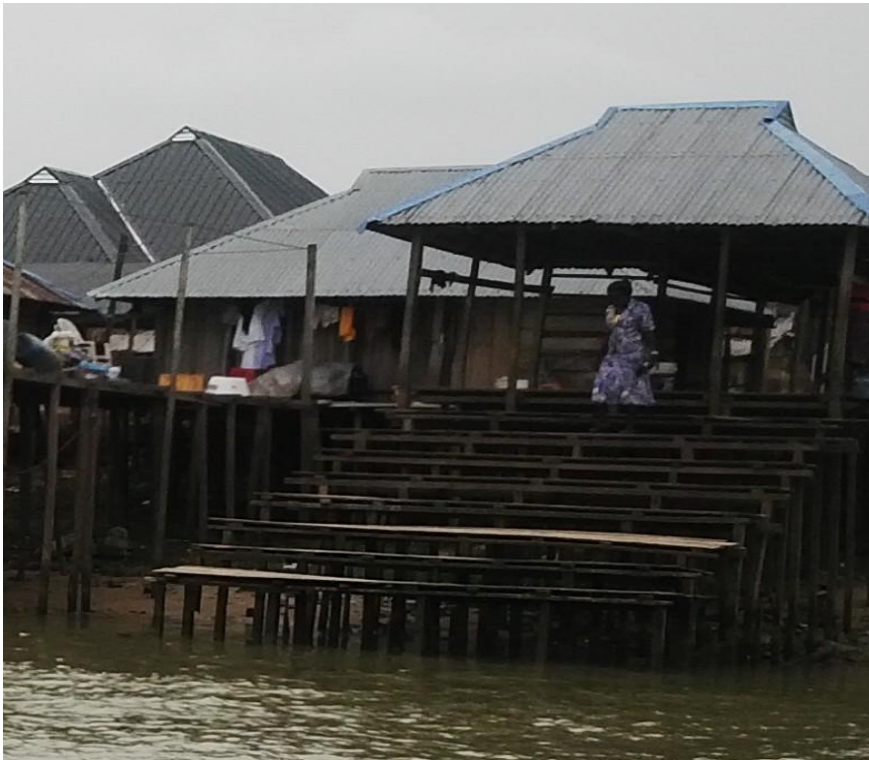
Plate 2: Harbour & Recreational Hall Stilt Structures using planks and zinc © O.K.Oyeoku & A.O.Angba
